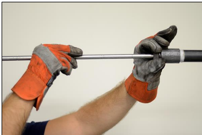
Figure 12 - Removing insertion rod from access port
