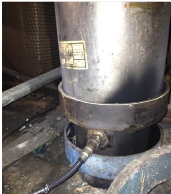
Close-Up of BIQ Sensor Installation with Top Exhaust
