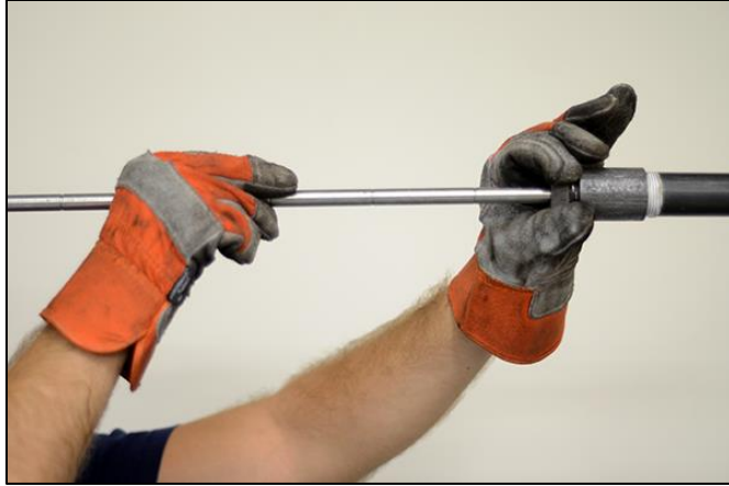
Figure 17 - Removing insertion rod from access port
